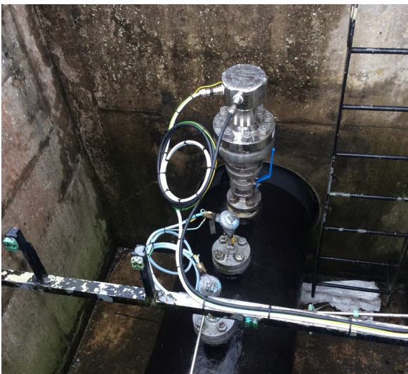
LineVu installation at a gas entry point to the NTS
